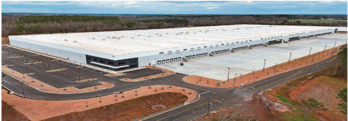
This warehouse in Social Circle, Georgia, is among the largest bought by the Trump administration in an effort to expand migrant detention spaces by converting facilities nationwide into huge holding centers. MEGAN VARNER/REUTERS
